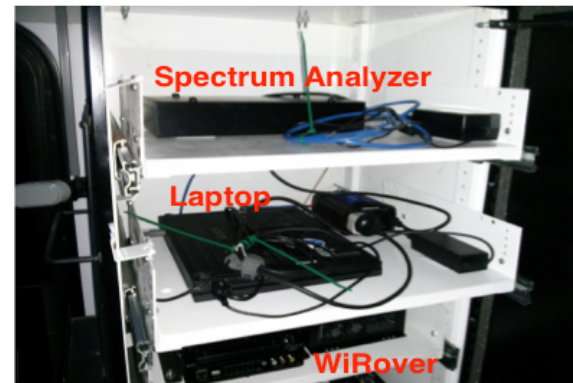
Cabinet inside bus
